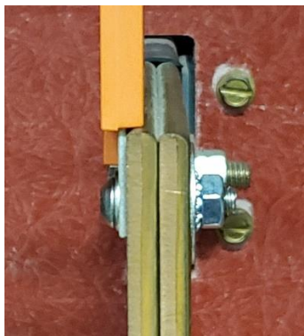
Figure 14: CC-TC sensor with nut and bolt mount cross section view
