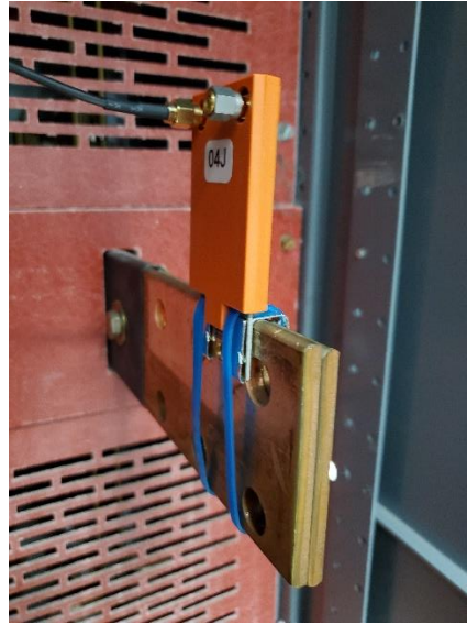
Figure 17: CC-TC sensor with clip-mount and high-temp plastic ties
