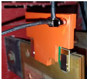
Figure 4: CC-WC wide-clip mount example
