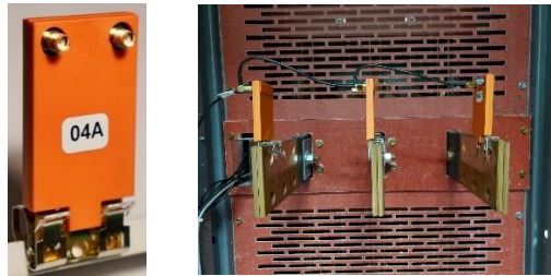
Figure 1: CC-TC single sensors mounting example on Air Circuit Breaker back lugs (right)
