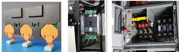
Figure 2: CC-E45 sensor module tie-wrap mount example on a MCCB (center) and fuse disconnect (right)
